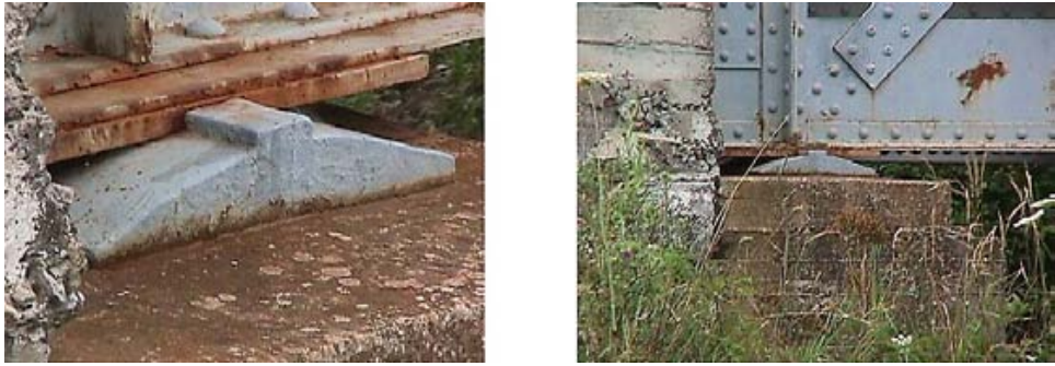
Fig. 6. Sliding bearing at end masonry piers.
