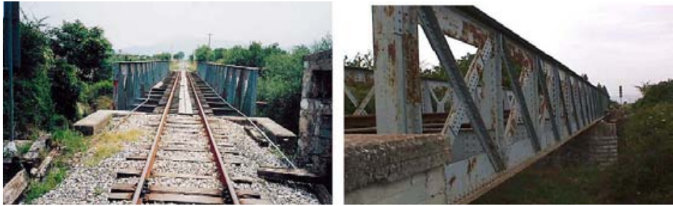
Fig. 1. General view of the steel bridge.
