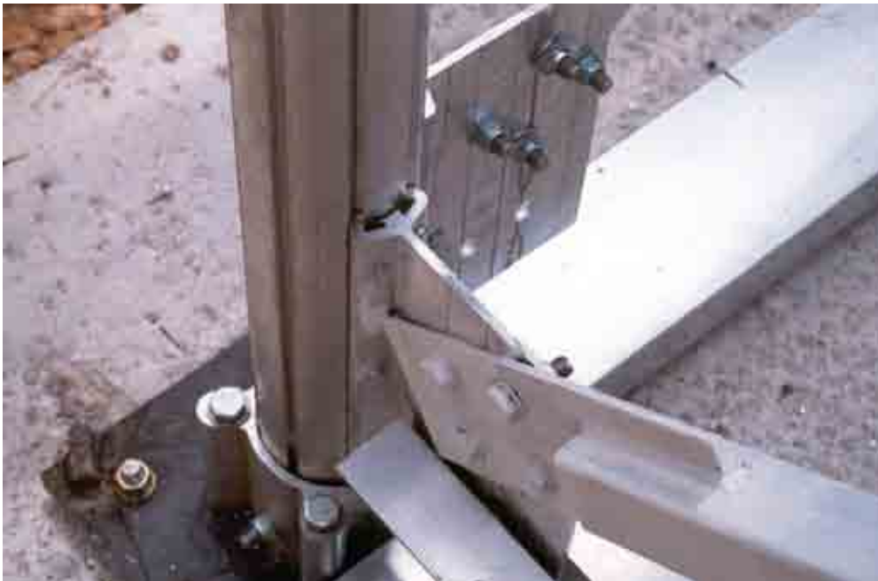
Fig. 9. Column–bracing–foundation connection.
