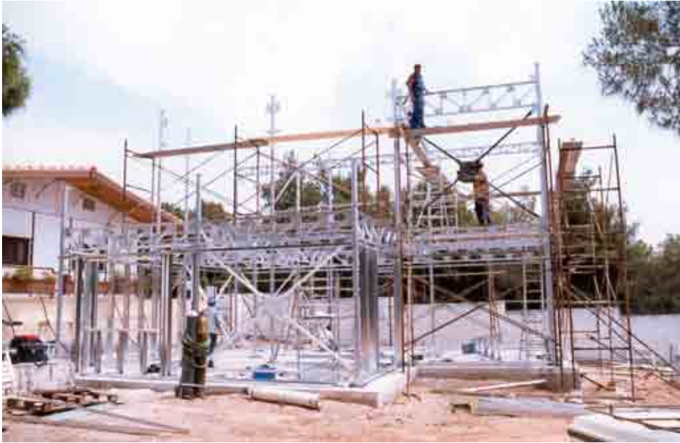
Fig. 1. Aluminum building frame under construction.
