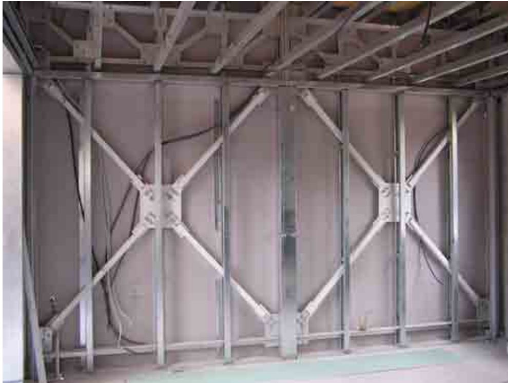
Fig. 5. Diagonal steel bracing.
