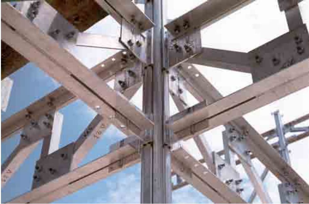
Fig. 8. Beam–column connection.
