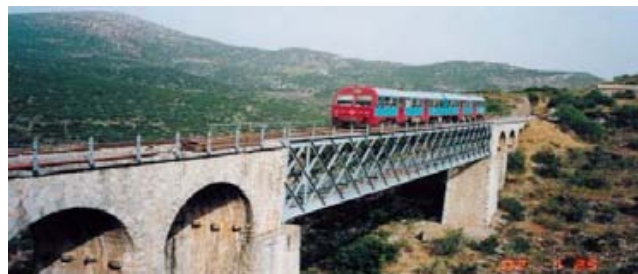
Fig. 1. General view of the steel bridge.
